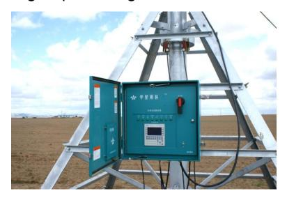
Workstatus showing, realtime monitoring, failure alarm, span body synchronization safety protecting function.
